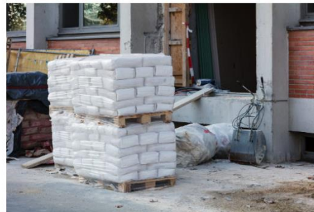
Bagged cement supplies for a house under construction
