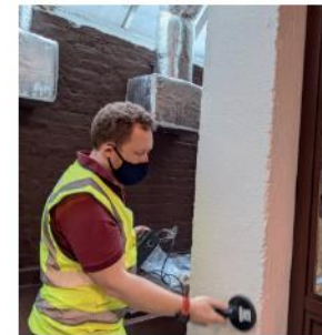
Using a metal detector to scan a concrete encased steel column at ground floor of 34 NR.
