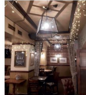
24 North Audley Street. Extensive finishes present within 24 AS. Beam down-stands obscured by ventilation boxing out.
