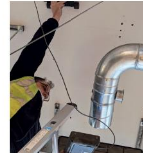
Scanning first floor of 34 NR using a cover meter.
